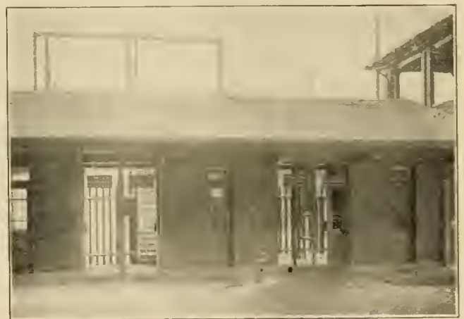
TIMEKEEPERS' BOOTHS AT MAIN ENTRANCE TO SHOP GROUNDS, FOR CHECKING THE EMPLOYEES IN AND OUT.
